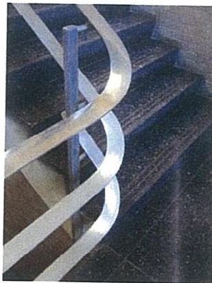
Wilber Hall - Central Stair
