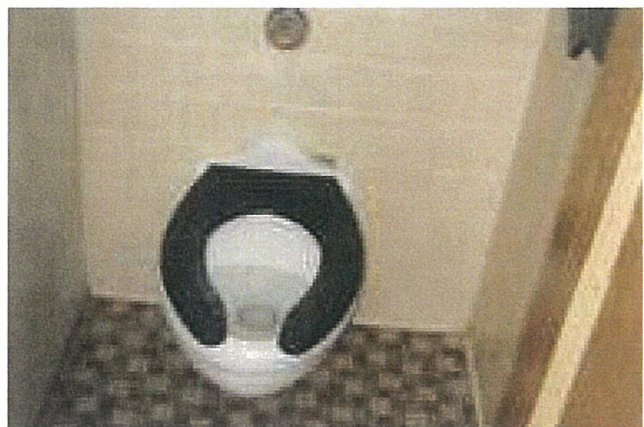
Wilber Hall - Toilet Room
