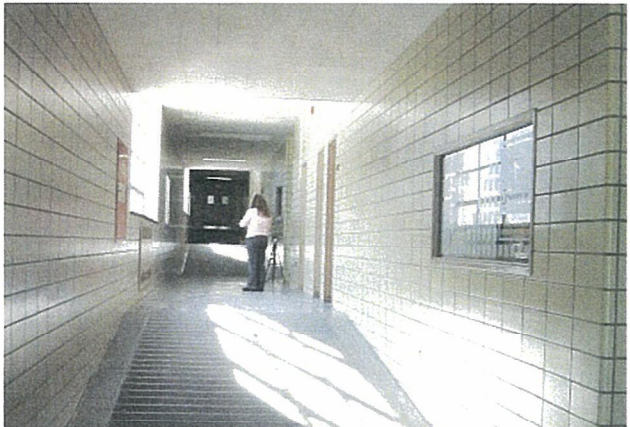
Wilber Hall - First Floor Corridor
