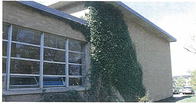
Wilber Hall - East Wall
