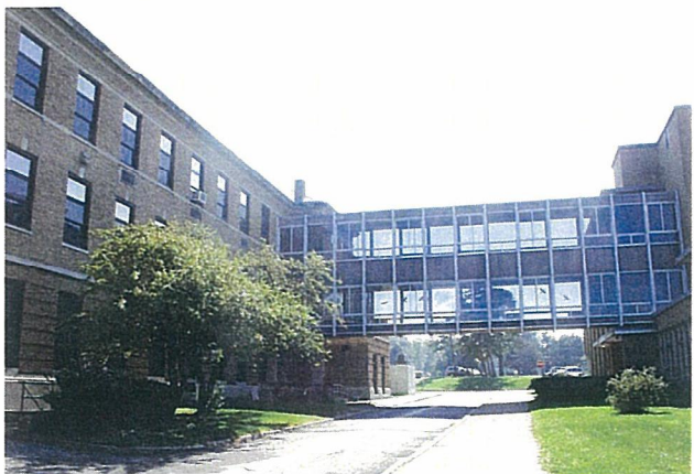
Wilber Hall -Bridge Link and Adjacent Site Conditions
