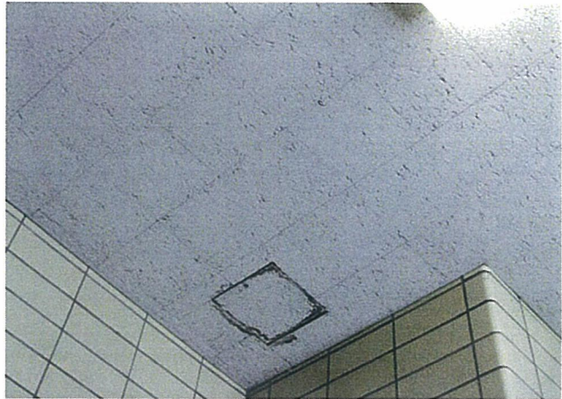
Wilber Hall - West Stair - Ceiling
