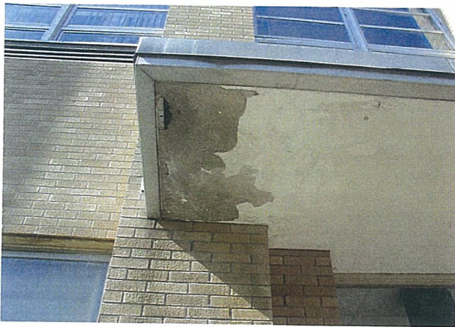
Wilber Hall - East Wall - Entry Soffit
