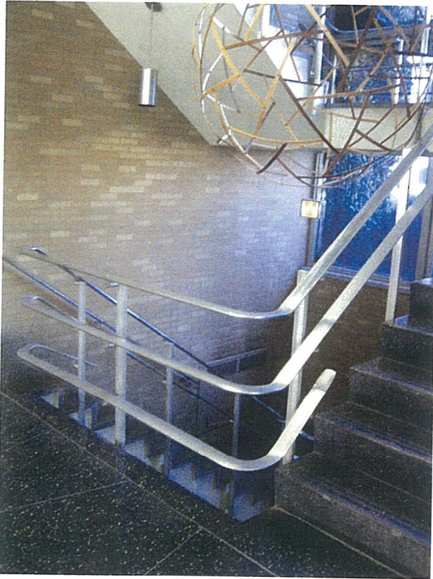
Wilber Hall - Central Stair
