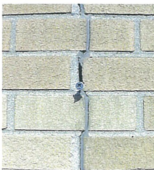
Wilber Hall - West Wall - Fifth Brick Pier
