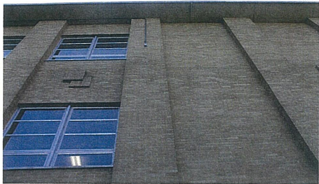
Wilber Hall - North Wall - Fourth Pier to the West
