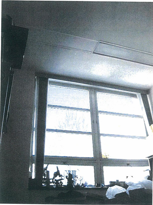
Wilber Hall - Room 254
