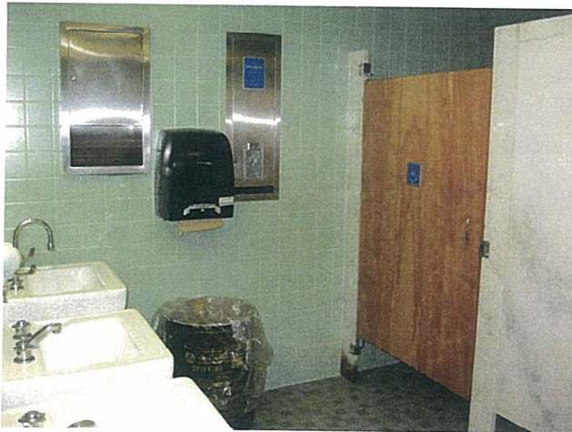
Wilber Hall - Women's Toilet - Second Floor
